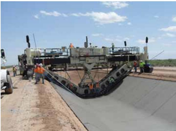
As an alternative to a custom built solution, G&Z's Highway and Airport Concrete Paving Equipment can be converted into canal and reservoir liners with minimal modification. The G&Z TC1500 can also be converted to a cure jumbo for canals and reservoirs.
